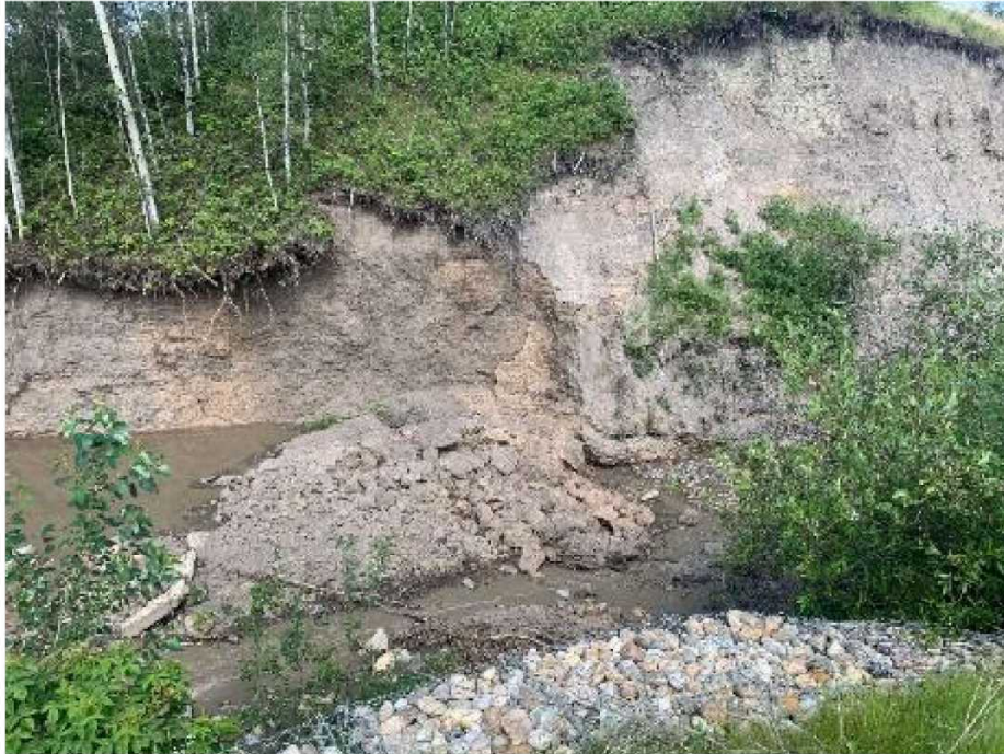
Photo 51: Partial blockage/damming of Bouffieux Creek due to debris failure on the inside bend adjacent to Old Fort. July 10, 2020
