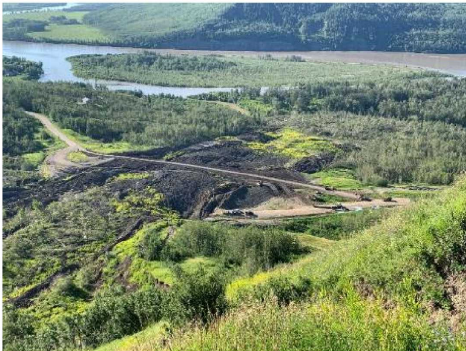
Photo 34: Temporary access road spans earthflow and began allowing 4x4 traffic into Old Fort. July 10, 2020
