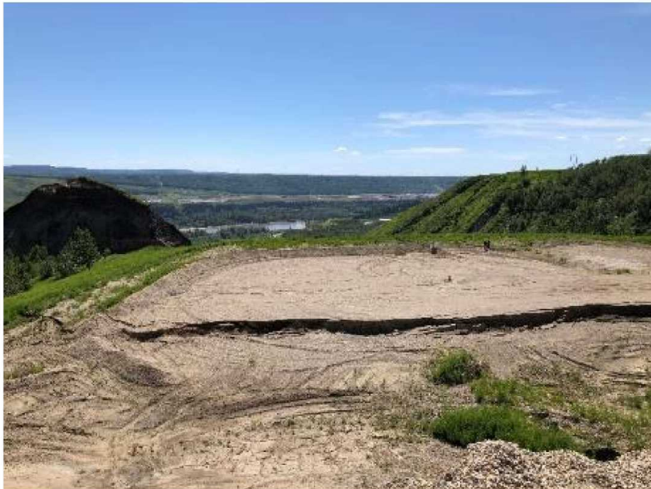
Photo 20: Large tension crack crossing the length of the lower borrow pit bench. June 24, 2020
