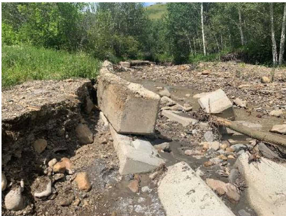
Photo 48: Additional failure of the concrete lock blocks in Bouffieux Creek east of Old Fort. July 8, 2020
