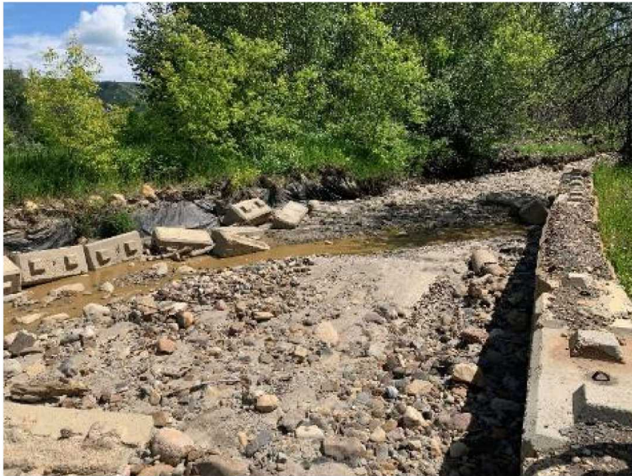
Photo 41: Lock block armouring (failing) east of Old Fort in Bouffieux Creek. June 22, 2020
