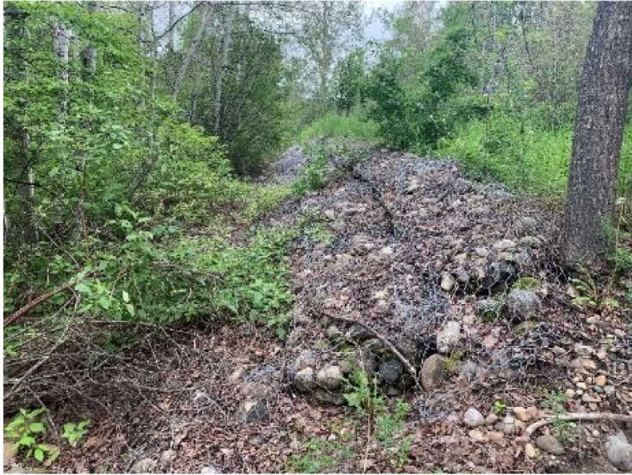
Photo 35: Gabion baskets at west end of Bouffieux Creek dike. June 22, 2020
