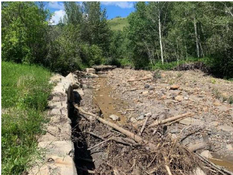
Photo 40: Lock block armouring (partially failing) east of Old Fort in Bouffieux Creek. June 22, 2020
