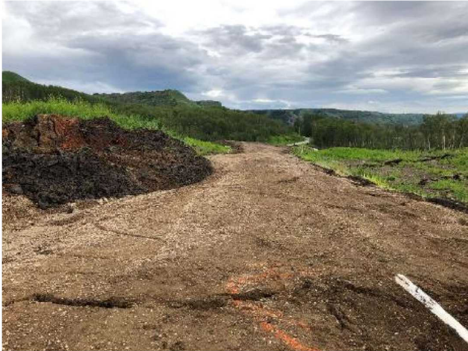
Photo 3: Old Fort Road being pushed to the south (note: tension cracks and earthflow bulge) June 20, 2020
