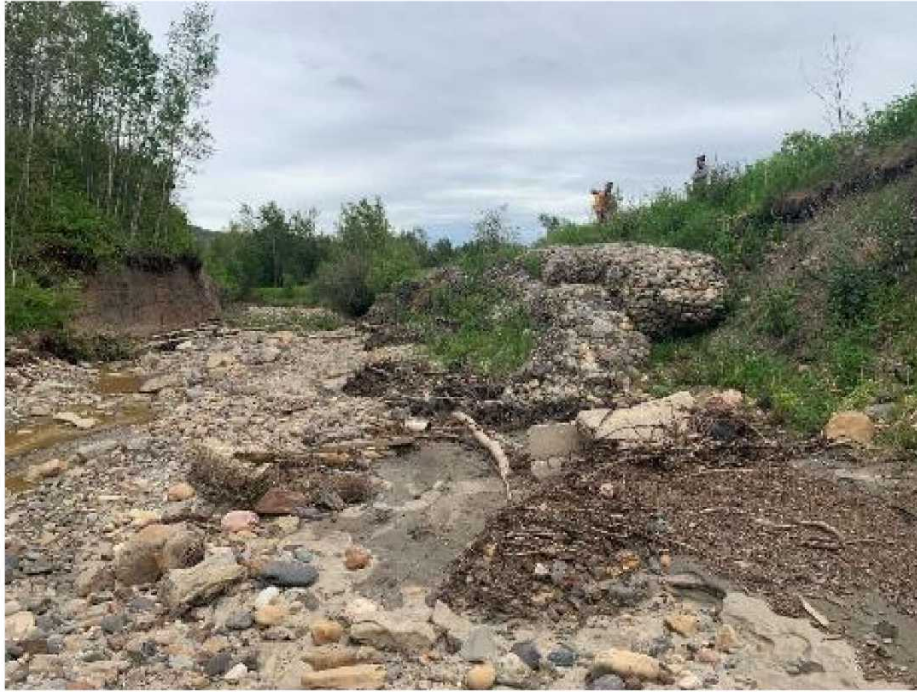
Photo 37: Gabion baskets partially in Bouffieux Creek near residential area (looking downstream). June 22, 2020
