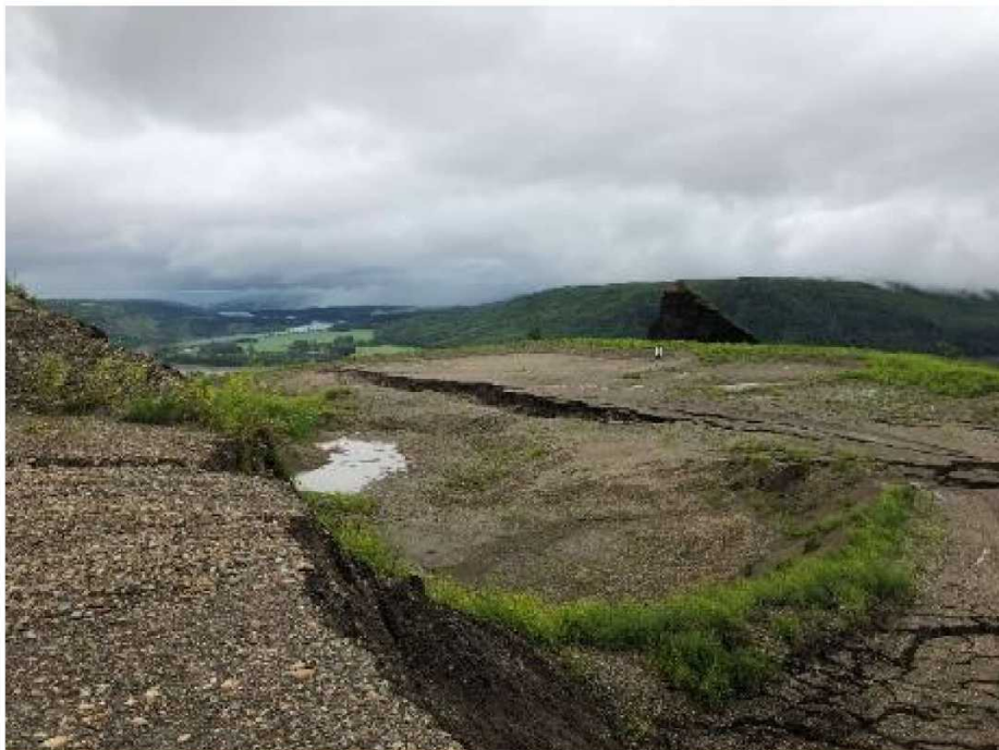
Photo 24: View of lower bench in borrow pit (tension crack trends approximately west-east) July 3, 2020
