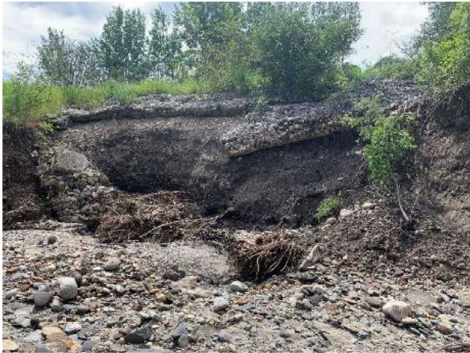
Photo 46: Bouffieux Creek bank and gabion basket failure (see Photo 38 for pre-storm picture). July 8, 2020
