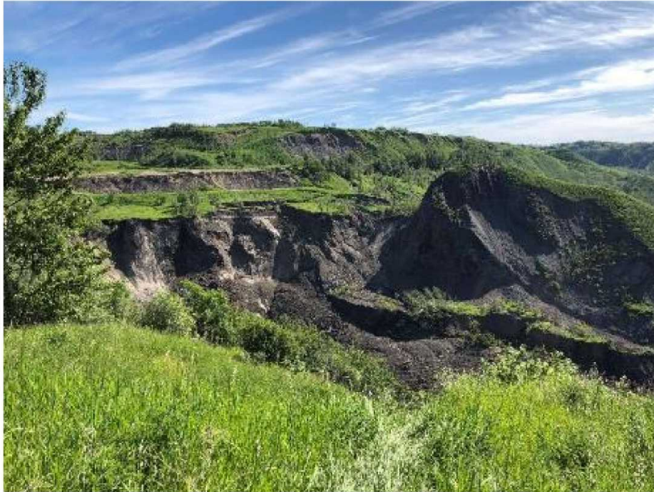
Photo 19: Overview of the back-scarp (borrow pit), main scarp (foreground) and ridge. Earthflow flowing left to right. June 24, 2020
