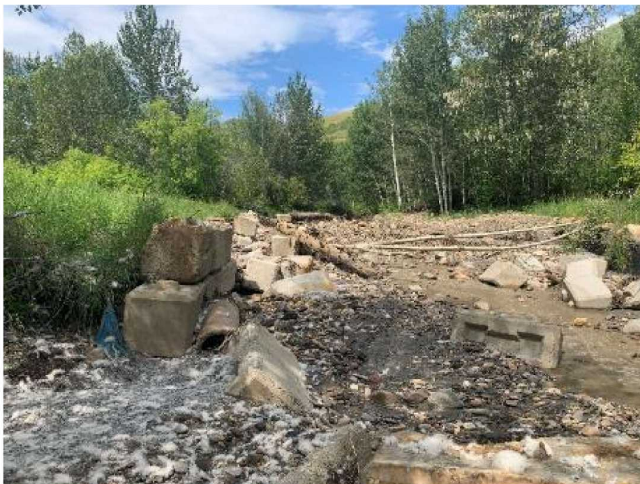
Photo 47: Additional failure of the concrete lock blocks in Bouffieux Creek east of Old Fort. July 8, 2020
