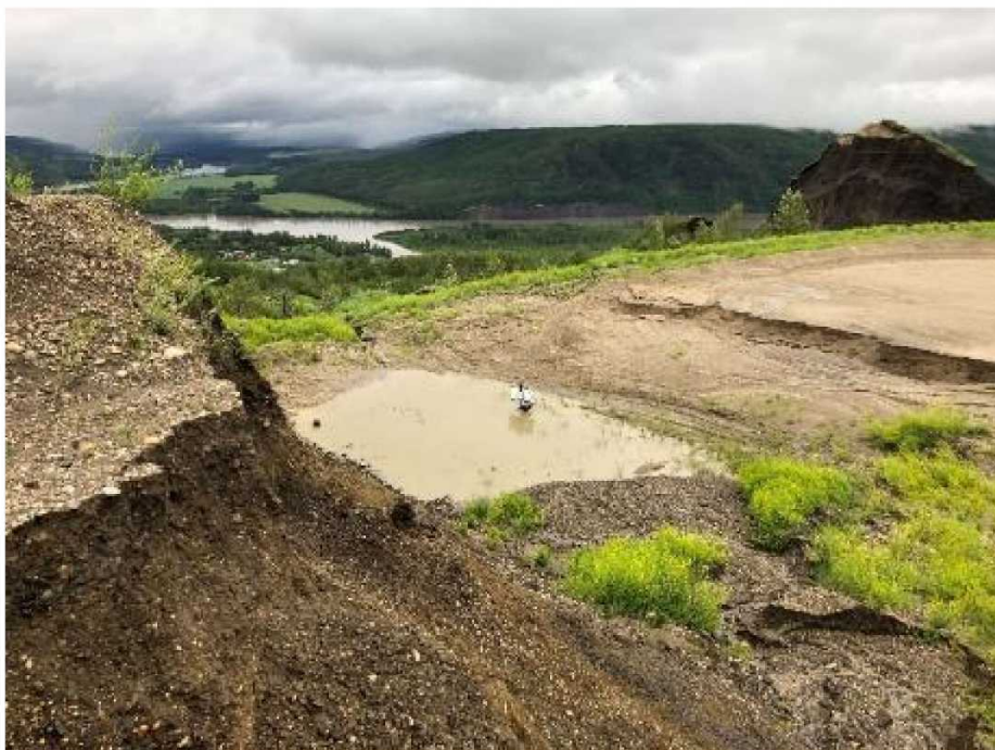
Photo 25: Pounded water in graben formed in borrow pit. MoTI GPS unit in pond around GPS unit. July 3, 2020
