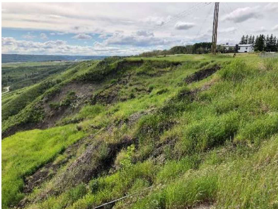
Photo 8: Slope relaxation and surface failures on the steep slopes on the south end of the look-out. June 20, 2020
