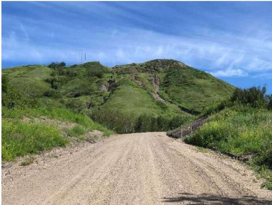
Photo 12: View of south facing slopes (below look-out). Multiple surface instabilities (shallow slump-flows). June 22, 2020
